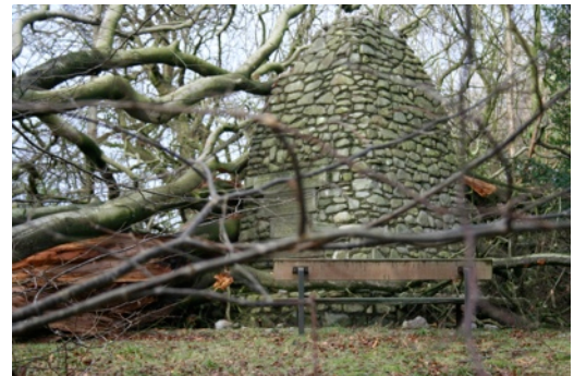
The Damaged Robert Burns and William Wallace Cairn.
